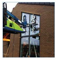
The Winlet 350TH has a hydraulic system which makes it independent from the telehandler.
